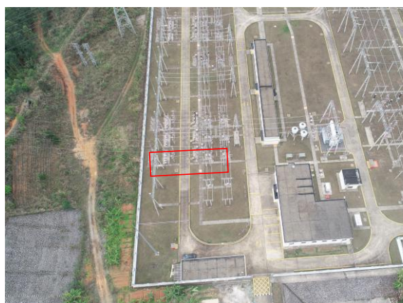
傍浦变电站扩建间隔
