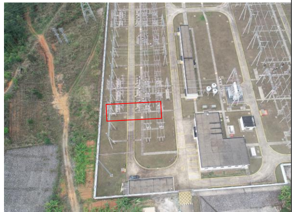
傍浦变电站扩建间隔
